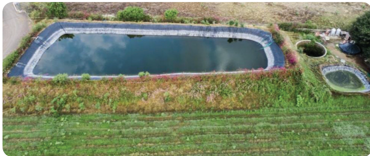
Ariel View of Rainwater Reservoir at Sula Vineyards
